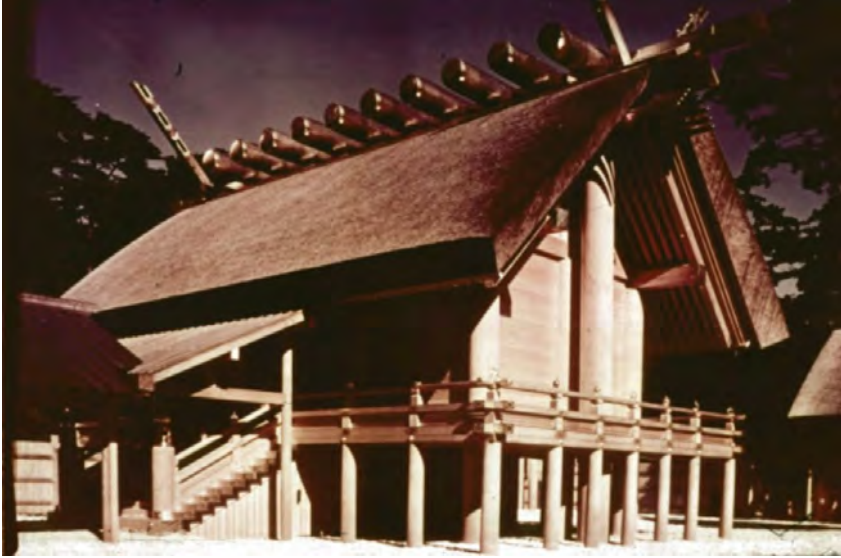
FIG. 16 Main Hall of Inner Shrine dedicated to Amaterasu, Ise Shrine, Mie Prefecture, Japan. Rebuilt every 20 years since the late seventh century.
