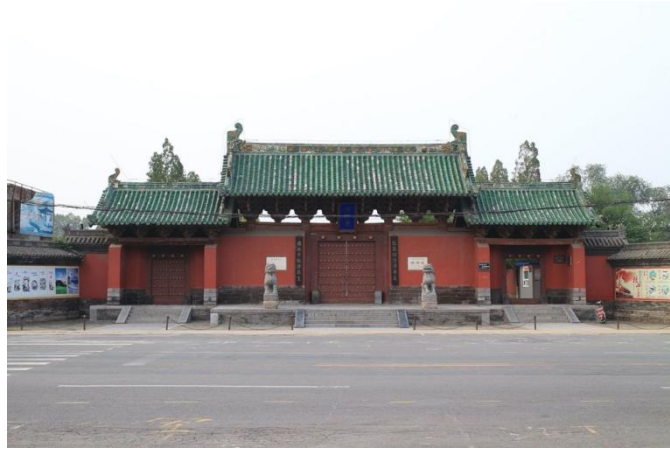
Figure 1 Front gate of the Jidu Temple (Gate of Pellucid Headstream Grotto 清源洞府門), photo by Li Teng, 2017.07.
